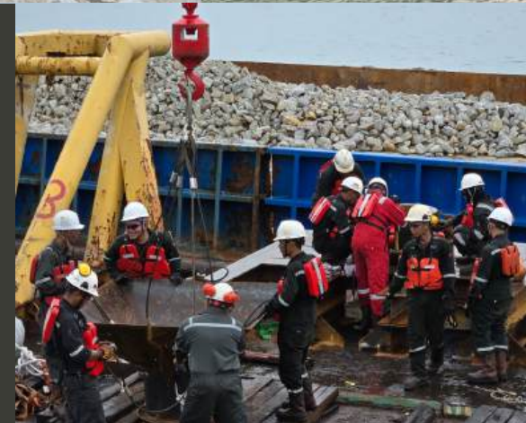
Funneling Rock Dumping on Seabed
